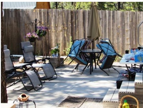
The New concrete patio with furnishings.
